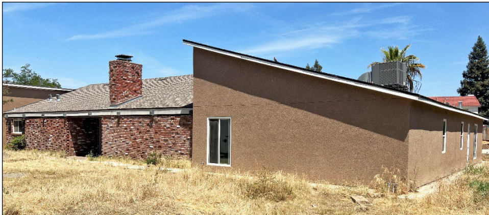
Façade and east elevation, view to the northwest (5/25/22).
