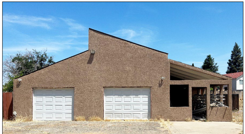
Garage, view north (5/25/22)
