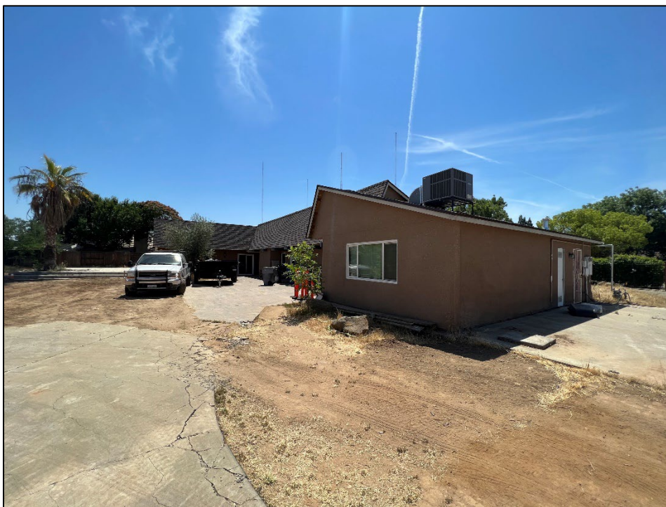
Photo 1: Northwest corner of house. Note various ground conditions. View southeast.
